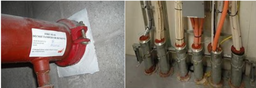
Figure 4: Fire Stopping Through Walls and Floors
